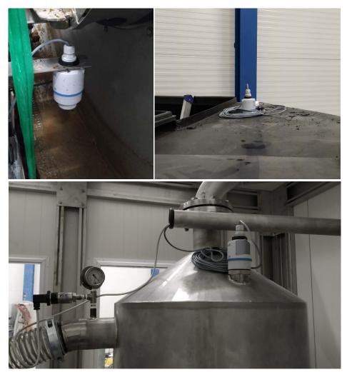
Figure 4: System sensors (top left) Level sensor in the sludge tank. (top right) Level sensor in the buffer tank. (bottom). Pressure sensors and level sensor in the vacuum taak
